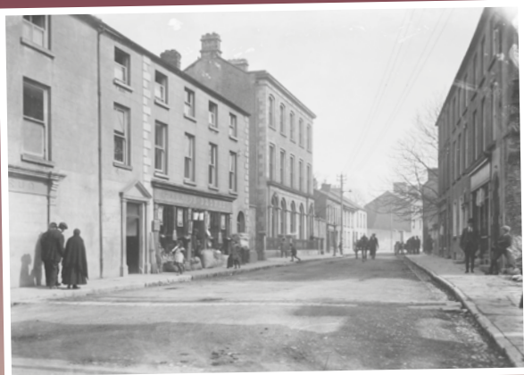
Dublin Road, Tuam
